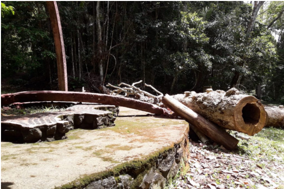
Figure 2. The damaged monument "500 years of Resistance by the Indigenous Peoples of Brazil" (Monte Pascoal, Bahia, 2020)
